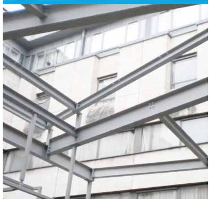
A centrally placed steel flitch plate was integrated with the existing steels in the building and was used as the main support for the rooflight, whilst the ten separate individually shaped sections of glass were secured off the steel spine using aluminium back to back angles. Even though it was a rigorous process, Glazing Vision's high level of precision and expertise ensured that the installation was carried out efficiently.
